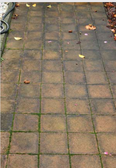
Moss and algae avoidance by reducing water absorption
