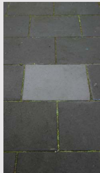
Absorption comparison 16 month after the application Single pavers treated.
